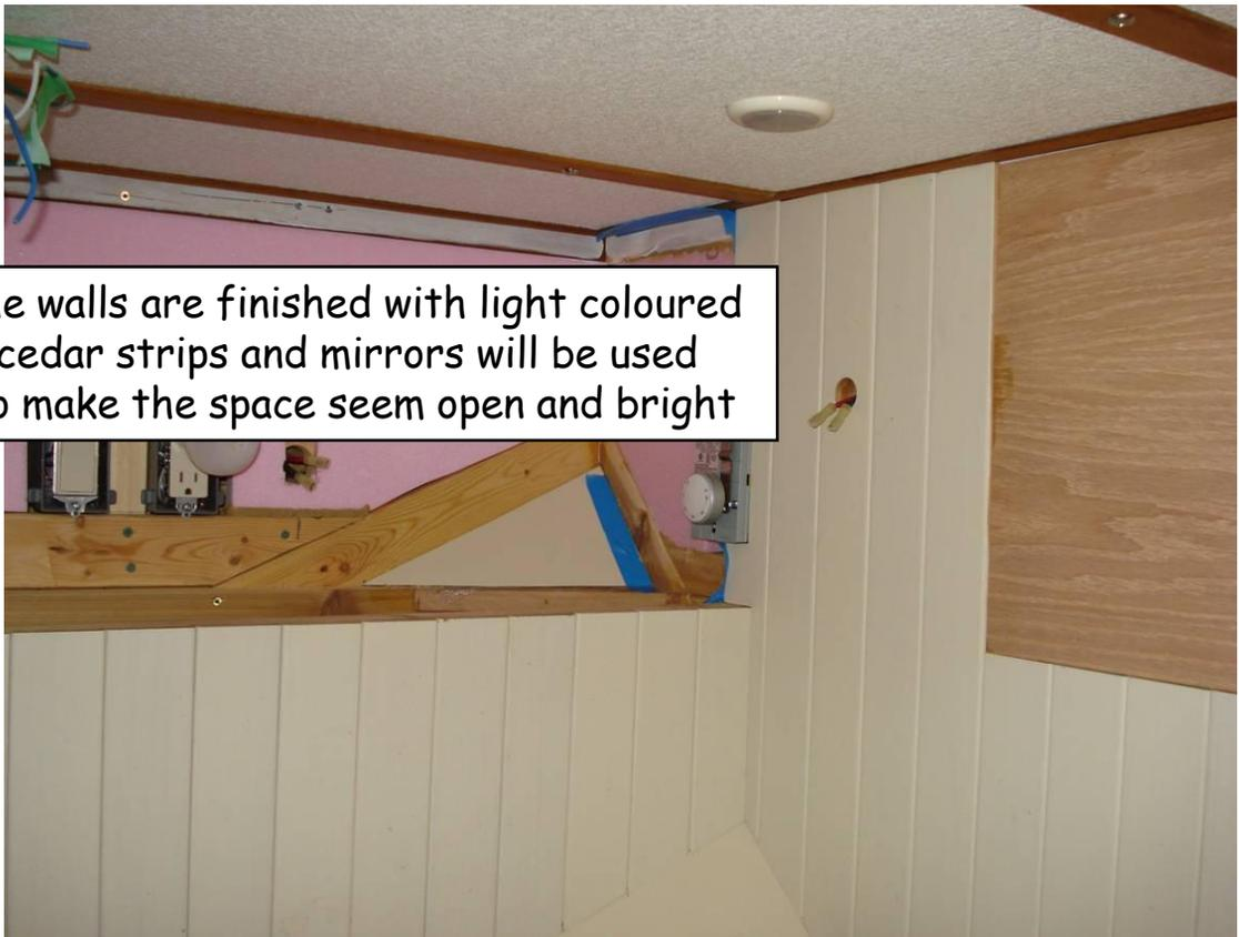
The walls are finished with light coloured cedar strips and mirrors will be used to make the space seem open and bright
