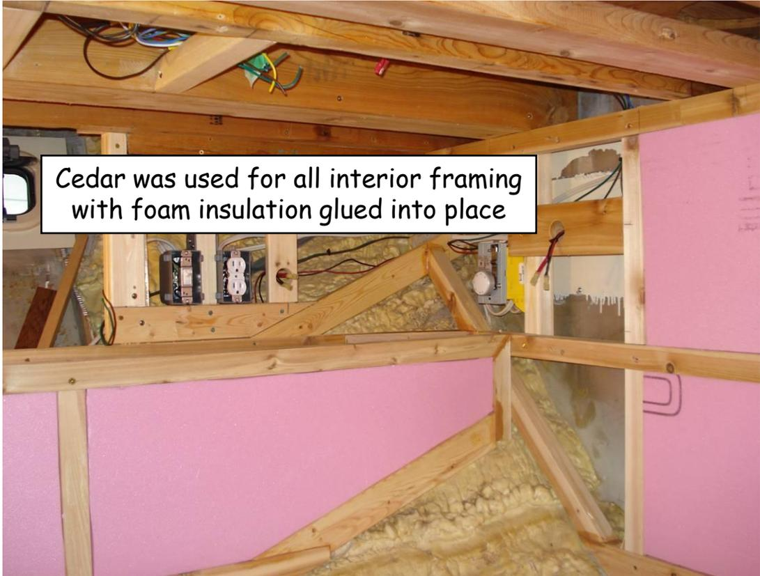
Cedar was used for all interior framing with foam insulation glued into place
