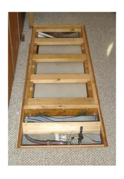
Originally, the new crosspieces were screwed into place above the tank. A subsequent modification was to make "pockets" along the longitudinal beams to set these into so that they are easily removable.
